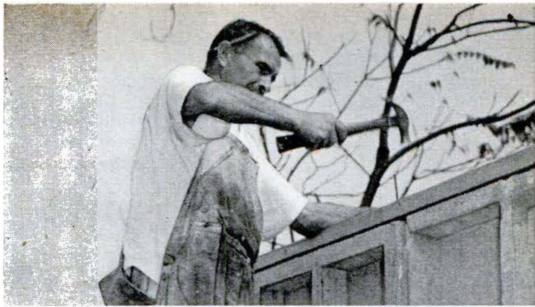
cast in concrete slab. Common wire nails can be hammered into the walls. Plates can be nailed or bolted to top of the walls.
